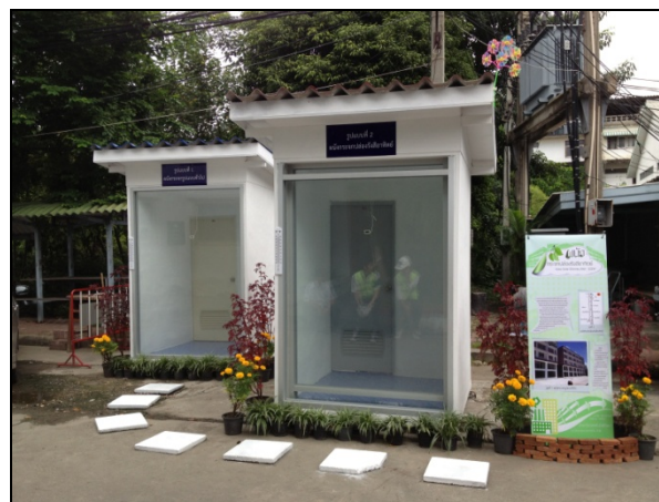
Fig. 3. OLGW and GSCW house for testing.
