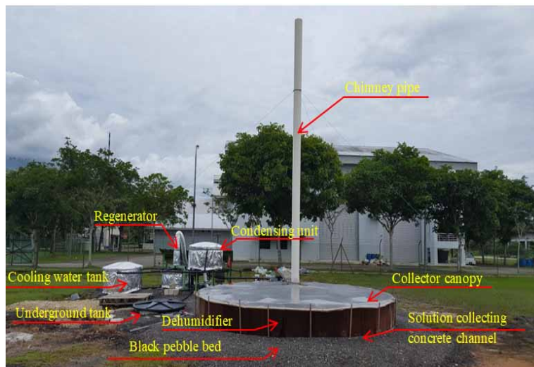
Fig. 5. Photograph of the pilot hybrid plant.
