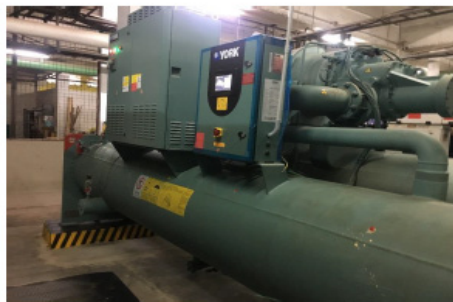
York Premium Efficiency VVWH 250 TR Water Cooled VSD Chiller
