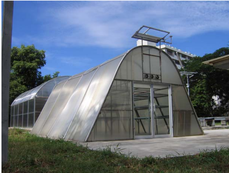
Fig. 1. Greenhouse solar dryer developed in this study
