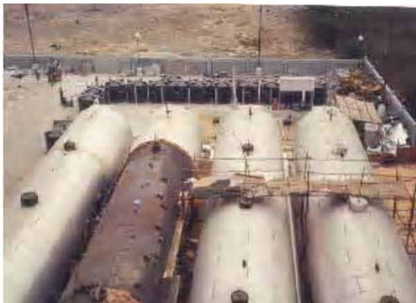
Fig. 4. Layout of 250 TR air-conditioning system integrated with CTES system
